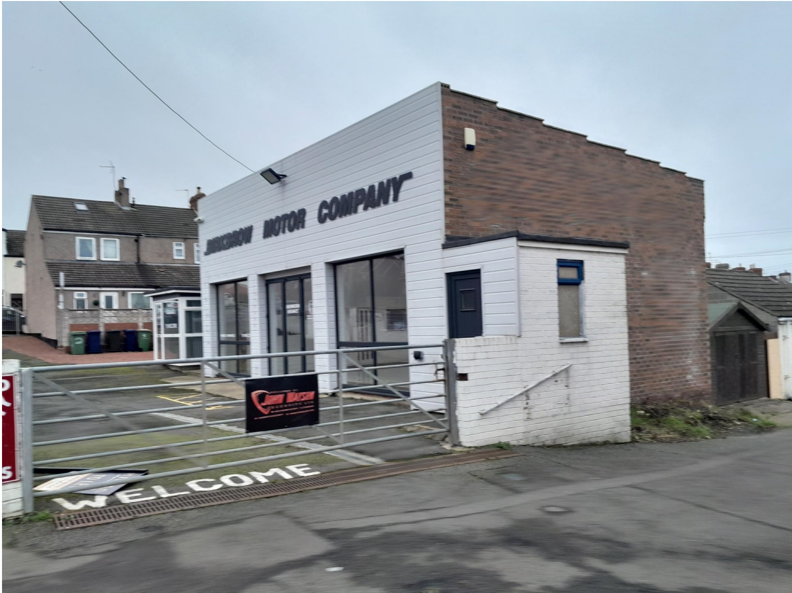
R/2023/0715/FF Liverton Mines Garage Photographs
