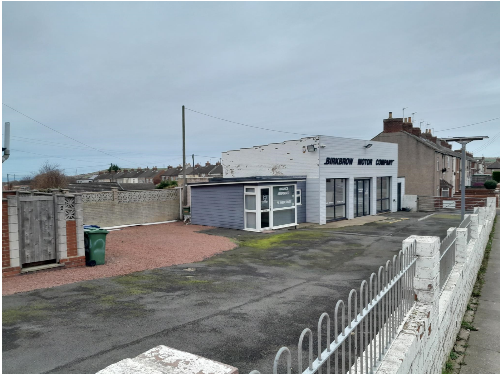
R/2023/0715/FF Liverton Mines Garage Photographs
